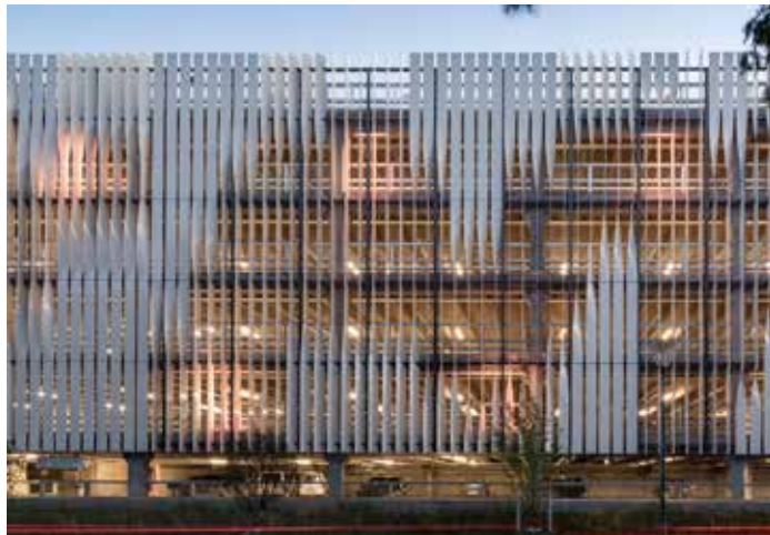
Future car parking Car park walls will be naturally ventilated and clad in high quality materials such as timber battens, or painted with large-scale public art murals
