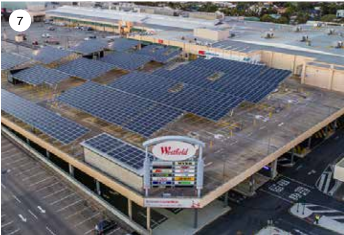
New Carpark Deck New parking will be provided for the increased GLA developed on the site in the form of new mezzanine parking levels. Photovoltaic cells are proposed on car parking shelters to provide shade and to offset part of the site's energy requirements.
