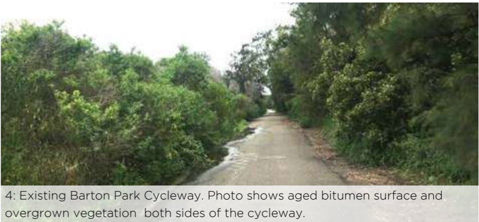
4: Existing Barton Park Cycleway. Photo shows aged bitumen surface and overgrown vegetation both sides of the cycleway.
